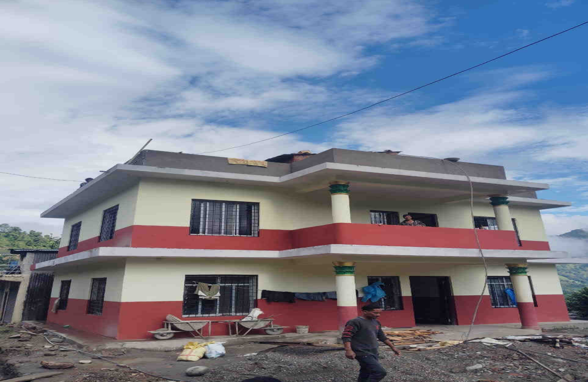
Adding 2 nd Storey Office Buidling in ward 4
