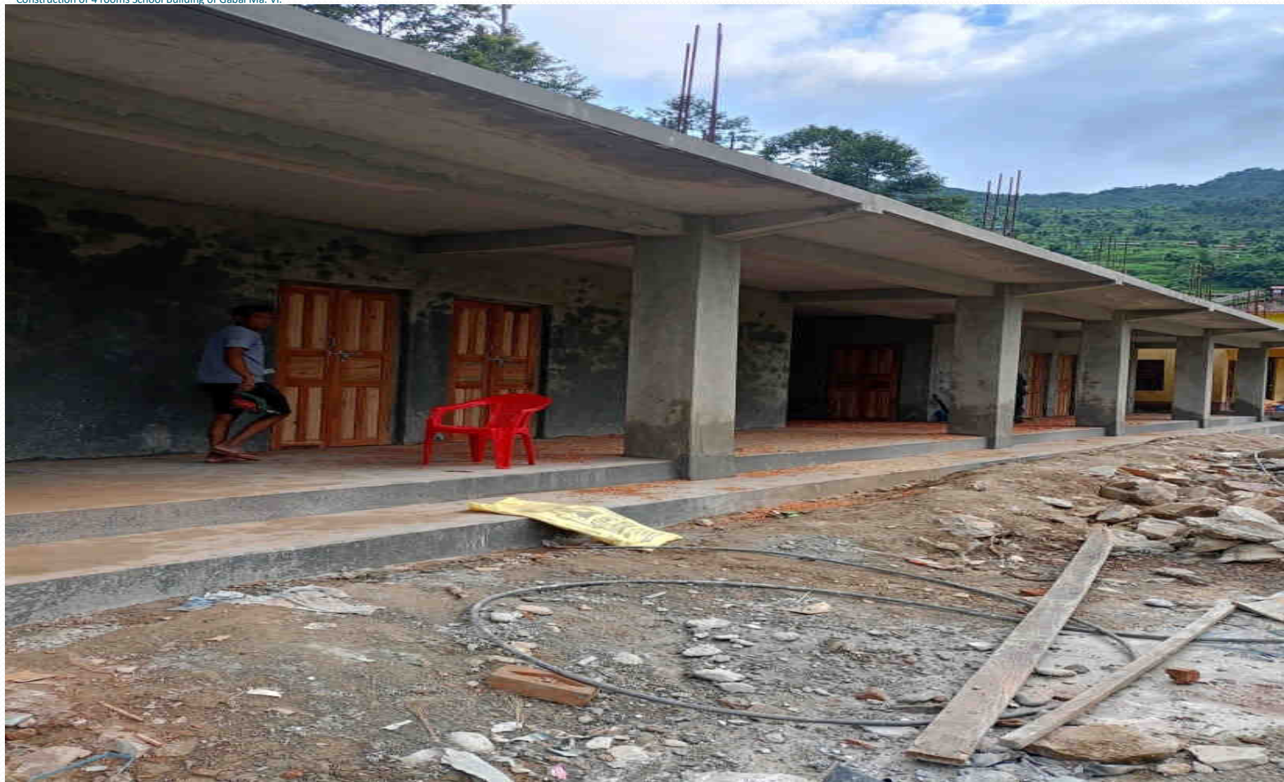
Construction of 4 rooms School Building of Gabai Ma. Vi.
